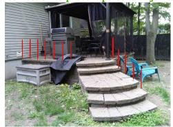
2. Grading: Negative slope observed - Negative grade slope noted on the Left, Right sides and rear. Immediate build up of positive grade slope (1 inch per foot for 6' from the foundation) is required to divert storm water away from the foundation and prevent water infiltration and damage to basement area.
