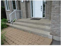
4. Marginal Deck: Paving stone - Safety railing missing around deck and steps, this is a safety issue that requires immediate correction to prevent personal injuries.
