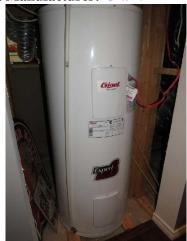
13. Type: Electric Capacity: 61.4 imperial gallons
