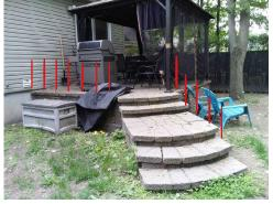
5. Marginal Grading: Negative slope observed - Negative grade slope noted on the Left, Right sides and rear. Immediate build up of positive grade slope (1 inch per foot for 6' from the foundation) is required to divert storm water away from the foundation and prevent water infiltration and damage to basement area.
