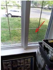
23. :2nd Floor Mezzanine Living Space Windows: Vinyl casement - Window fogging and moisture presence between glass panes noted due to damaged seals. Repairs required.
